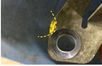
In this photo the area has been notched out and the bracket is fitted.
